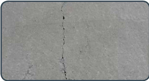
Despite adopting good design, detailing and construction practices, such as control joints and reinforcing mesh, to minimise the risk of cracking, there will be situations where cracks may occur as a result of movements in concrete due to changes in its moisture content and temperature.
