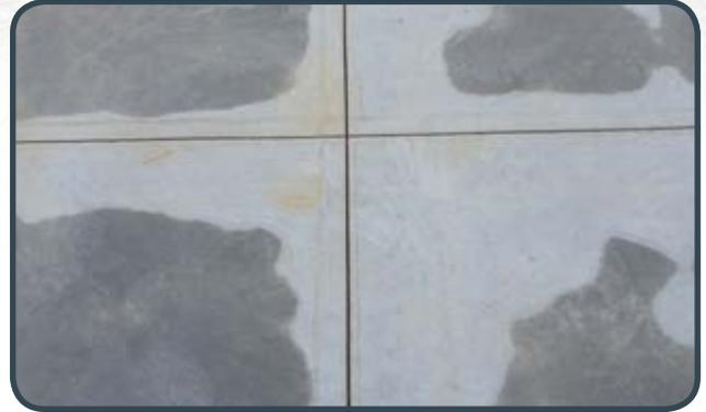
Letting the concrete weather may reduce the contrast in colour but does not always produce satisfactory results. Various proprietary applications are also available to mitigate the appearance of pinto.
