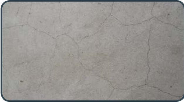
Cracks wider than 1mm should be assessed on an individual basis in terms of possible effects on durability and performance requirements and, depending on the surface texture and finish, also on aesthetic requirements.
