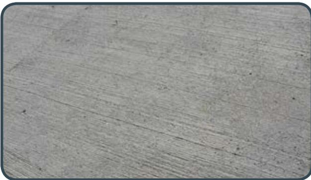
Sample panels can be used to agree on the surface appearance. The NZ Standard for concrete finishes requires sample panels to be viewed from a distance of 3 metres. View the driveway from this distance when assessing the driveway's surface finish.
